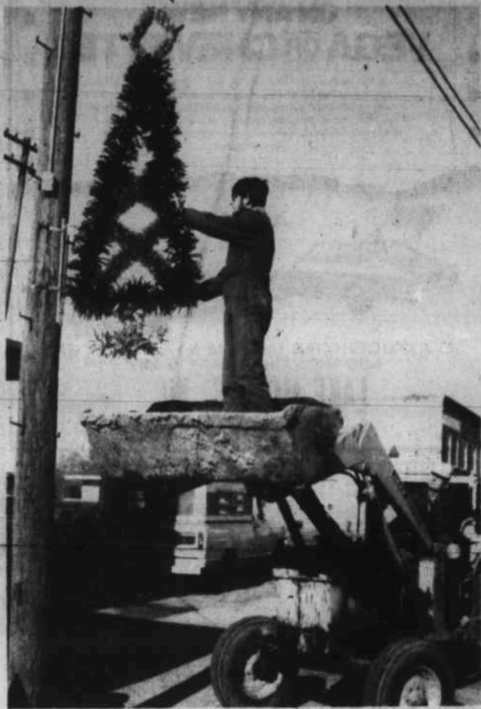
City employees Harry Supak, driver of the front-end loader, and Paul Supak are shown installing one of the new Christmas Decorations which will add beauty to the downtown area during the forthcoming holiday season. There will be 25 of the Christmas tree ornaments shown above and 25 candle ornaments and fixtures used at the Municipal Building will be refurbished under a program sponsored by the Chamber of Commerce through donations from local individuals and businesses.
